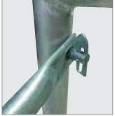
STEEL CROSS BRACING SECURED WITH ANTILUCE
